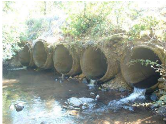
Reach 2 - Unit 187 5 Culverts in a row
