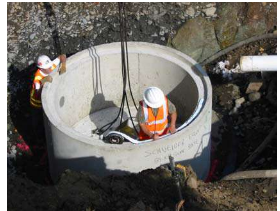
Following excavation the cylinders that comprised the pump vault were lowered into place.
