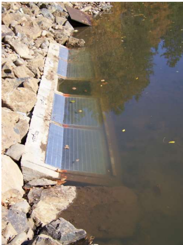
Photograph 11: Northeast from PP2 during re-establishment of the north bank following installation of the fish screen and pump vault (10/03/08).
