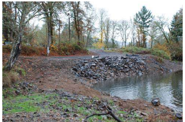
The north bank was restored to its previous configuration and re-armored with rip-rap.
