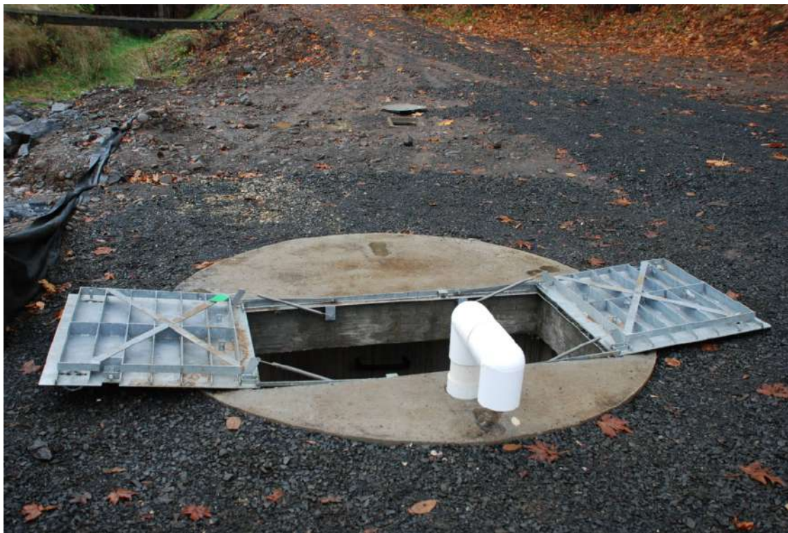
Photograph 16: View west at pump vault with doors open. Note small flowmeter vault with cover off near top middle of photo (11/11/08).
