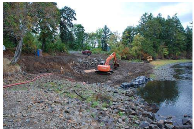
Erosion controls included straw waddles, silt fences, and an isolation dam (above).
