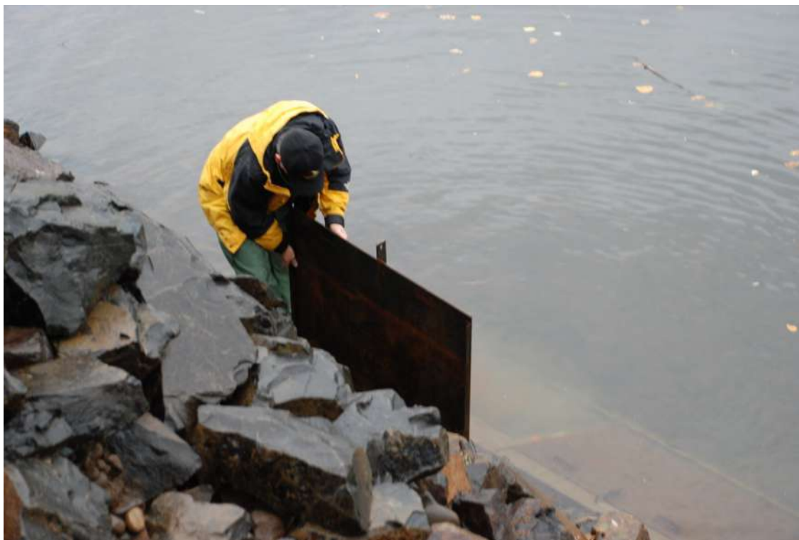
Photograph 18: View east from north bank during removal of fish screen cover plates prior to system test (11/11/08).
