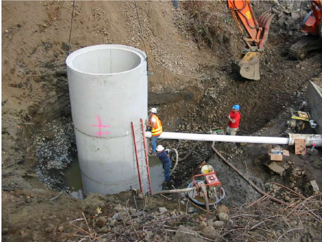
Photograph 9: View east at installation of pump vault and pipe from intake structure (on right) (9/26/08).
