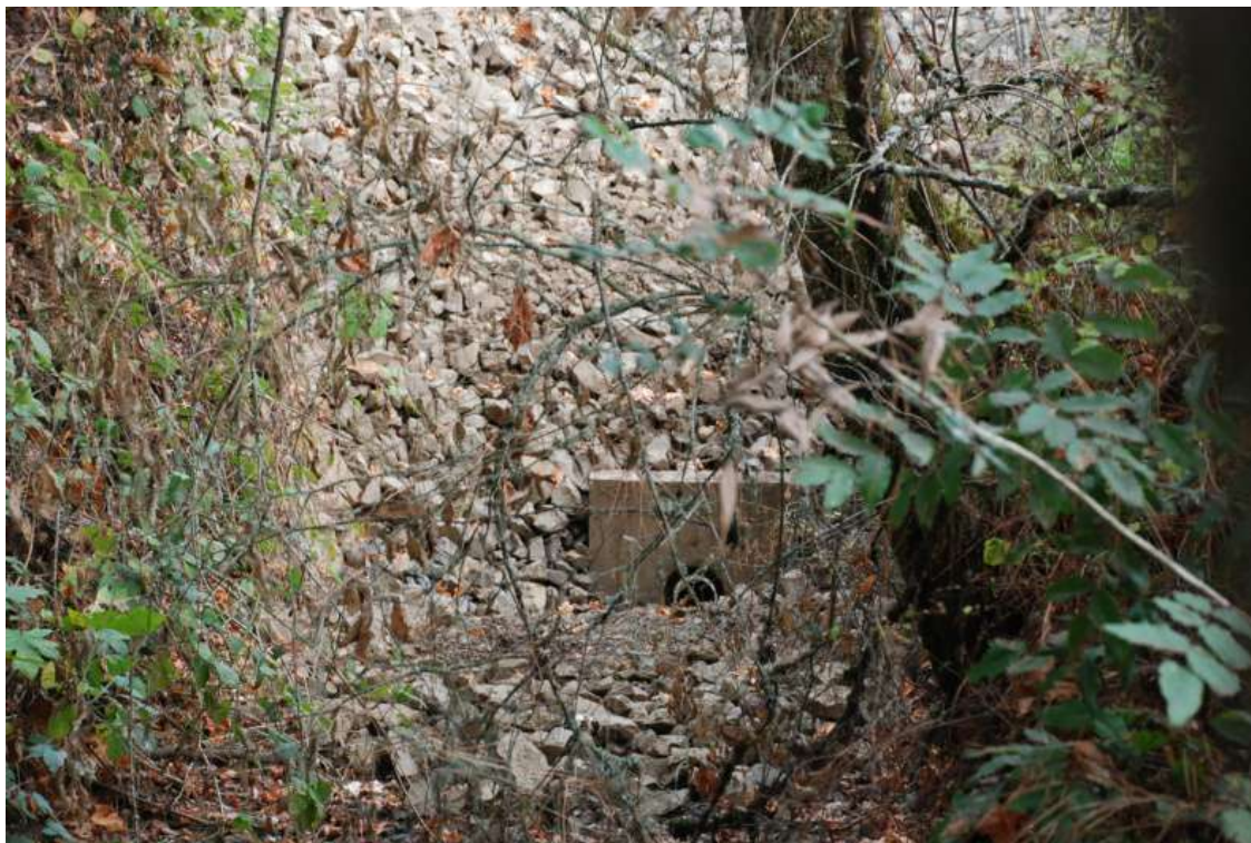
Photograph 14: View east at the completed dissipation structure in the canal with soil and rock berm above the structure (10/15/08).
