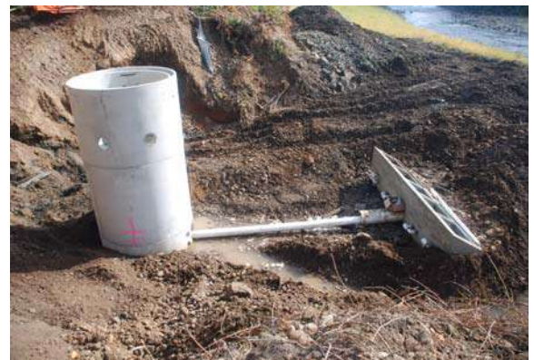
The irrigation diversion is a gravity-fed pump station with a fish screen over the intake.
