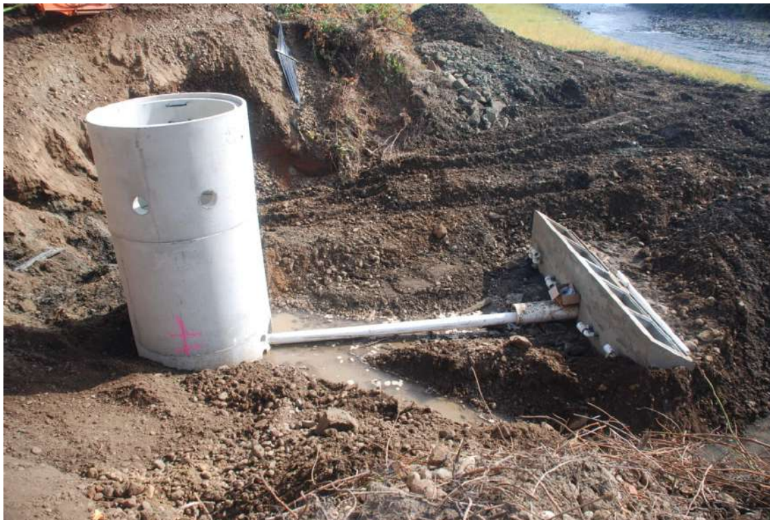
Photograph 10: View east at pump vault, pipe, and intake structure (9/27/08).
