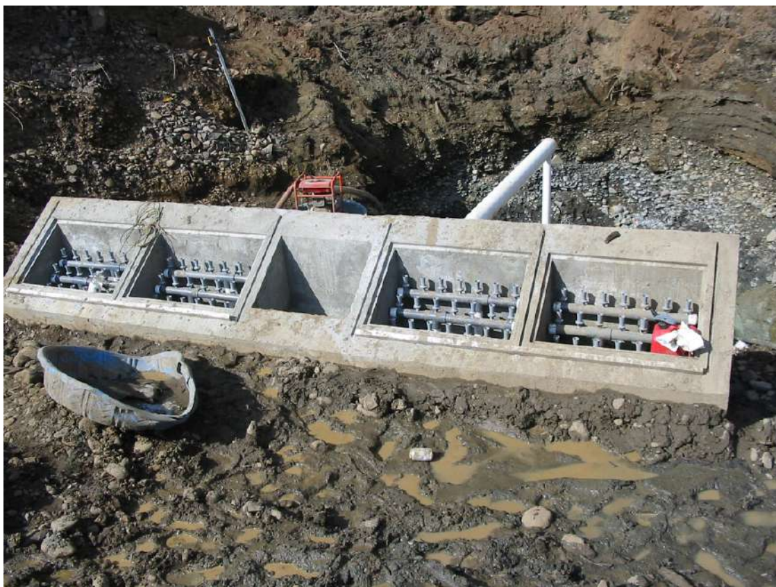
Photograph 8: View north at intake structure with fish screen cleaning jets installed (9/26/08).
