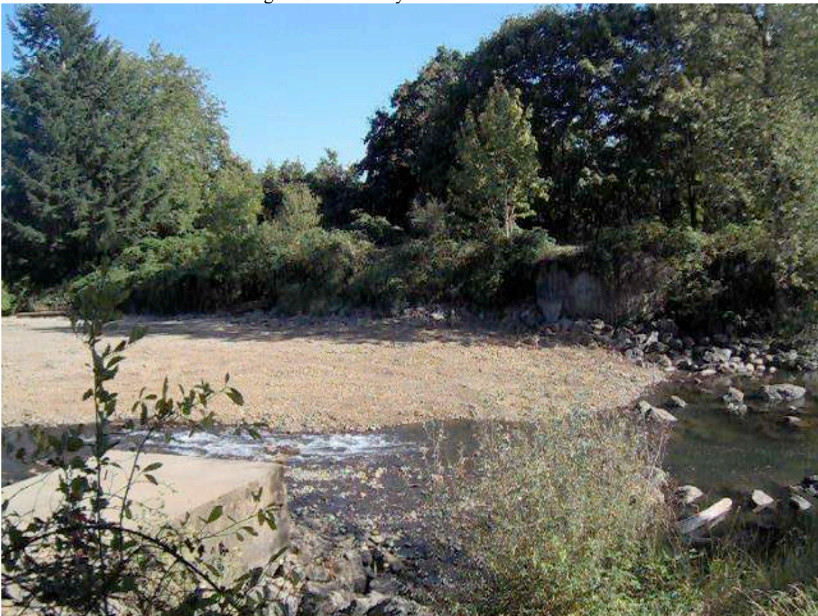
Brownsville Dam September 10, 2007 Entire dam removed. Abutments were left in place to provide bank protection.
