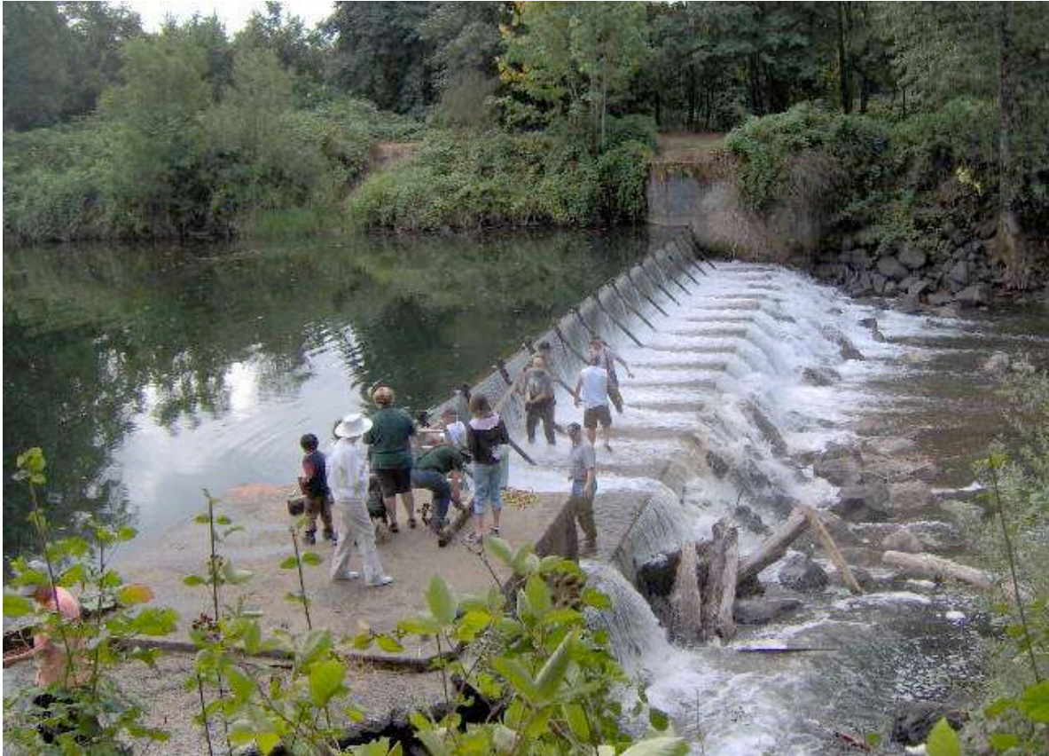
Brownsville Dam – August 18, 2007 Community members remove the flashboards for the final time. The flashboards raised the height of the dam by 5 feet to divert flow into the Brownsville Canal.
