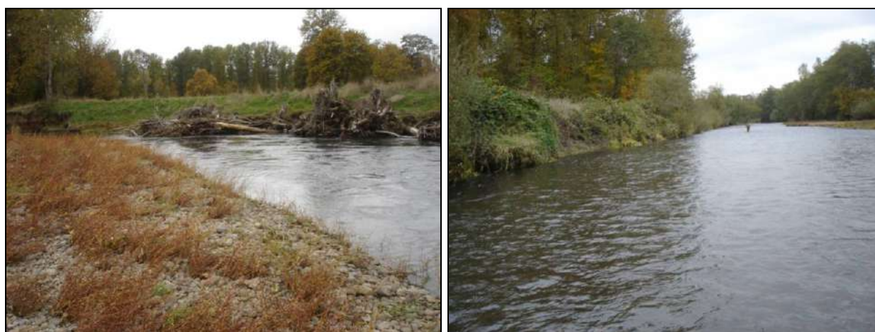
Figure 4-8. Examples of bank stabilization in Reach 3 include the Ross site (left) and an older riprap project spanning 2,000 ft from Sta. 242+00 to 262+00 (right).
