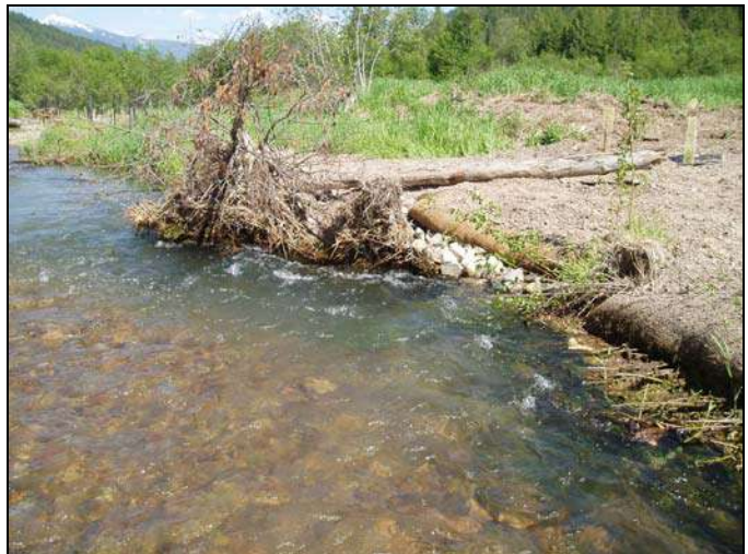
Figure 5-4. A large wood habitat composite with adjacent soil lift on Pilgrim Creek in western Montana.
