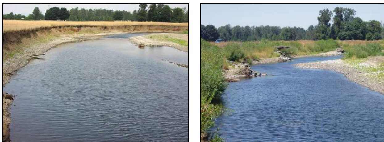
Figure 4-1. Examples of eroding bank (left) at the Carbajal site pre-project and more recent (right) photo showing effects of bank stabilization using rock barbs and revegetation.
