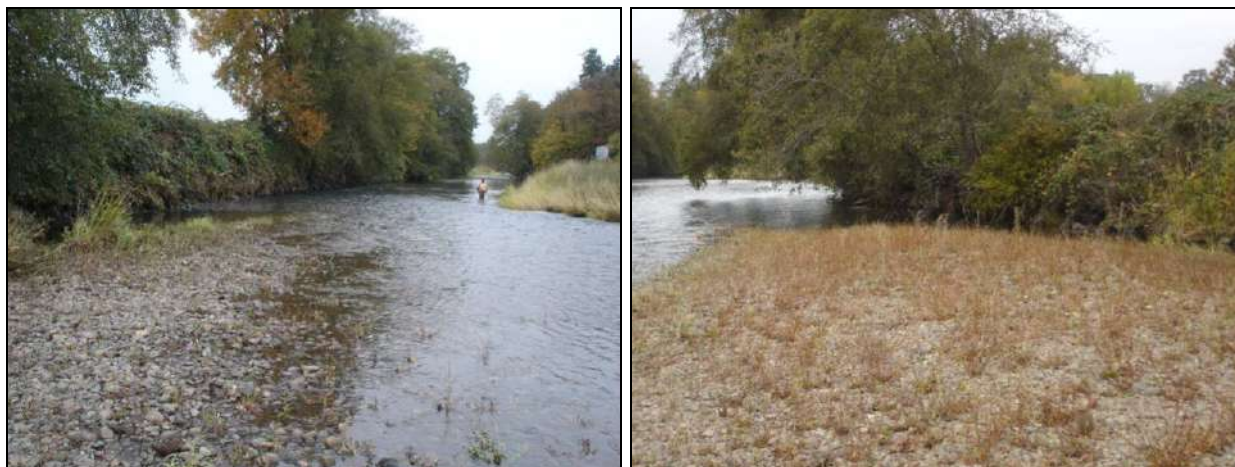
Figure 4-12. Examples of bank stabilization in Reach 4. The left bank is stabilized in upper Reach 4 (left). Blackberry bushes and deciduous trees have colonized the riprap. The right photograph shows a backwater habitat that has formed between a gravel bar and the adjacent riprap bank at station 309+00.
