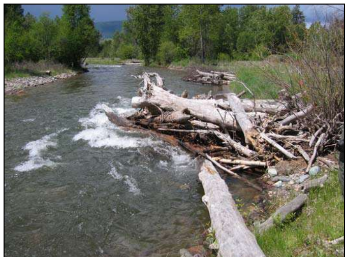
Figure 5-2. An ELJ constructed on the Jocko River in western Montana following two run-off events.
