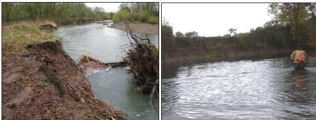
Figure 4-13. Example streambank failures in Reach 4 include the Smith property (left – photo courtesy of T. Putney) and the bank at Sta. 354+00 (right).
