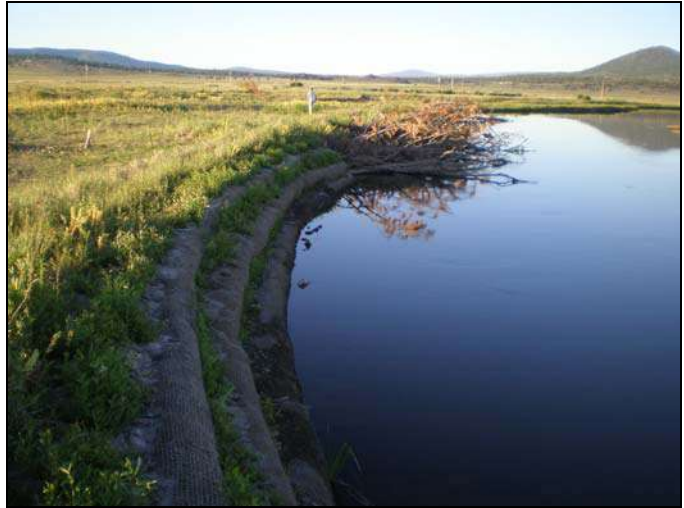
Figure 5-3. A vegetated soil lift following spring runoff and at the start of the growing season on the Sprague River.
